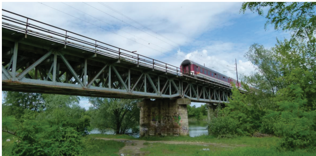
Figure 1. Sideview of a riveted truss bridge in Trnovec nad Váhom (Slovakia).
